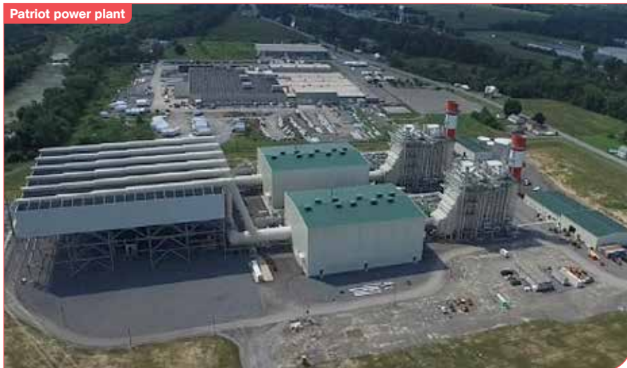
Patriot power plant
